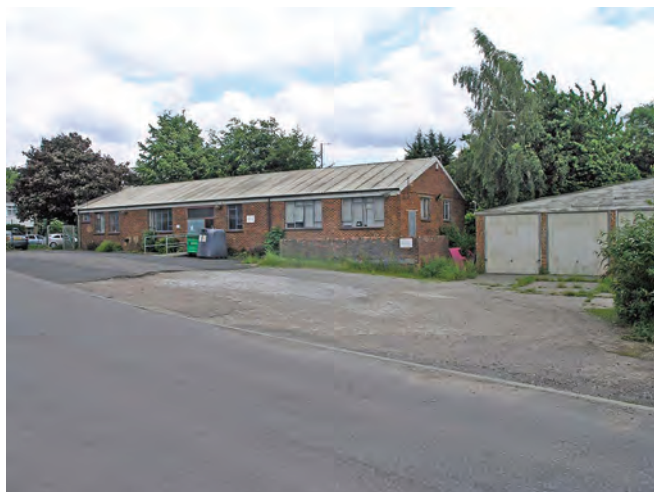
Training Centre at Vale Road, Northfleet. Civil defence ambulance garages are on the right
